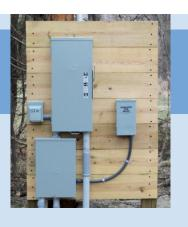
A transfer switch is a critical component when using a backup generator, as it prevents power from flowing back through the meter, transformer and onto the power lines. If a customer's generator sent power back onto the line, it could injure or even kill linemen who are making repairs to the line.
